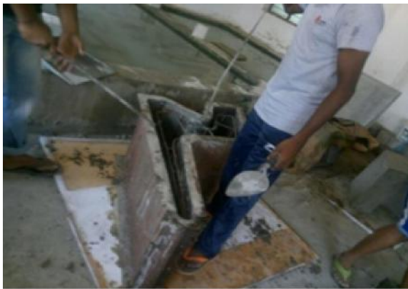
Fig. 3.21 Mould with rebar & mesh
