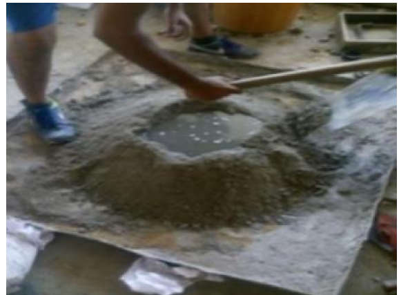
Fig. 3.20 Activated mortar
